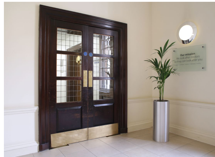
Doors leading to the corridor of the Carter and Worcester rooms when accessed from lift no.8
