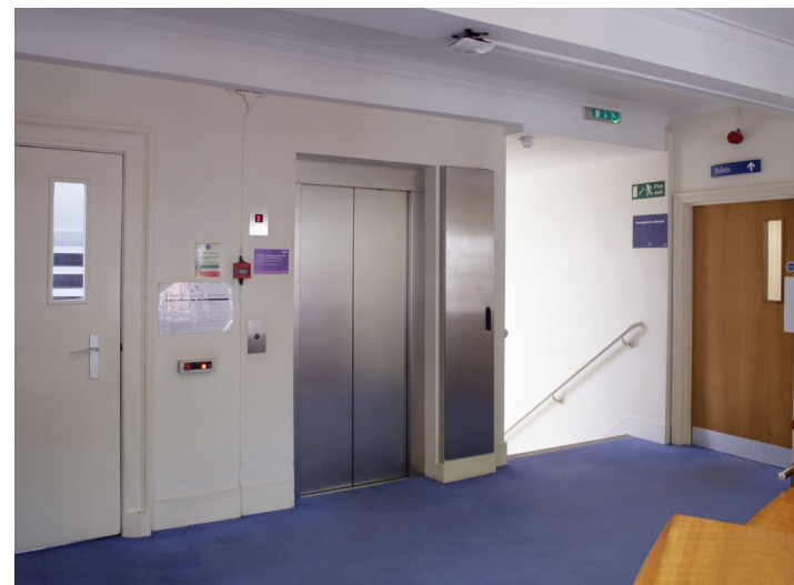
Lift no.11 – third floor
