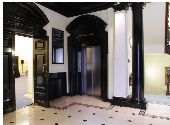
Lift no.3 – first floor
